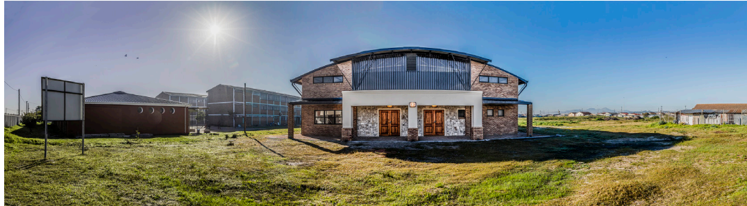
Chris Hani Arts and Culture High School Archway Foundation Hall in Khayelitsha
