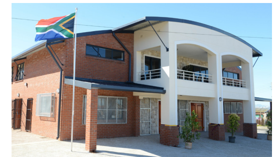
Sullivan Primary School Archway Foundation Hall in Steenberg
