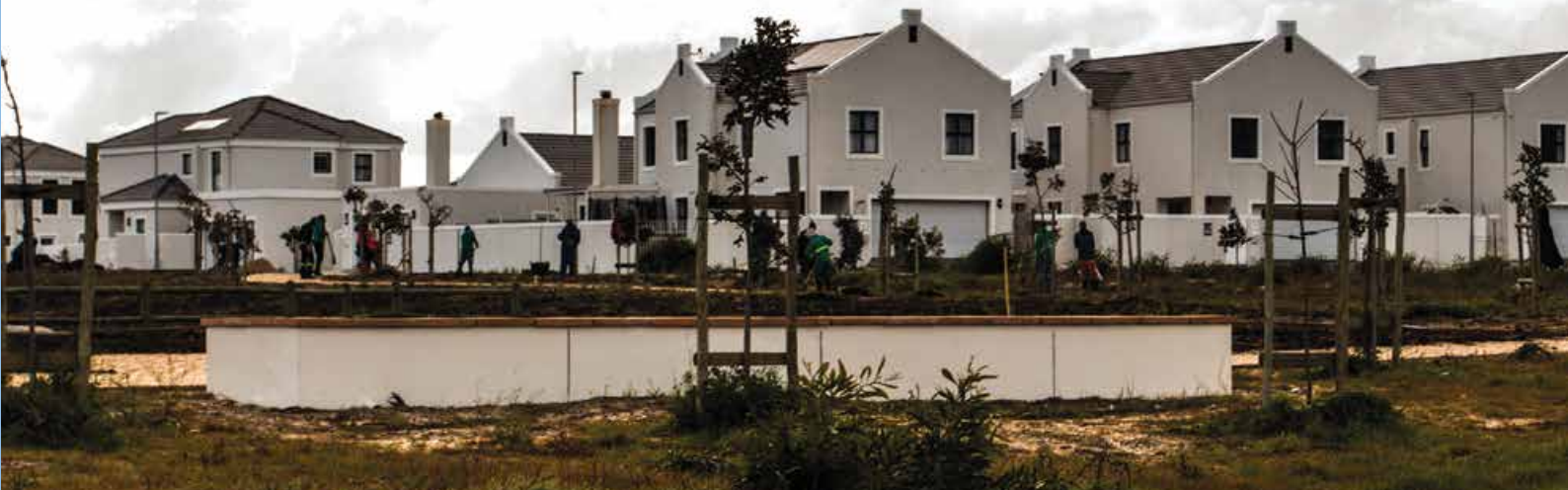
Sunningdale - extensive landscaping practices underway.
